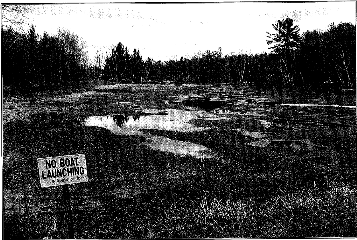
Figure 5. Five foot water level drawdown at the Beecher Lake Dam.
